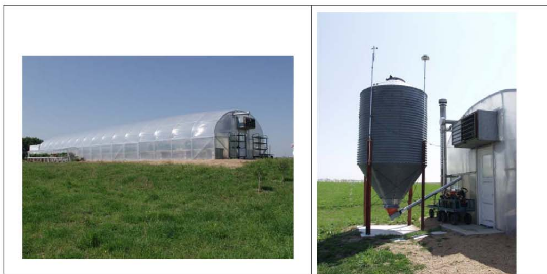
Figure 1. (Left) Commercial Greenhouse used in this study (Right) Corn storage bin and biofurnace flue pipes (Note the outdoor pyranometer and wind speed sensor at top of the bin).
