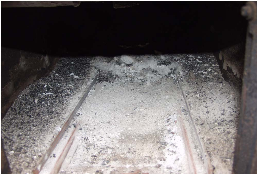
Figure 3.6. Firebox Ash Buildup.
