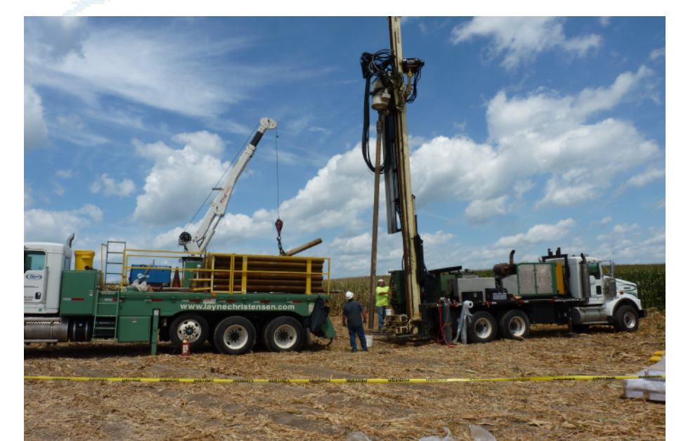
Figure 17: Deep Core Sonic Drill.
