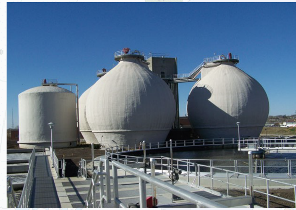
Figure 4: Theresa Street Wastewater Treatment Plant Lincoln, NE. Pictured are large anaerobic digesters which have the capacity to facilitate methanogen growth and biomethane production.
