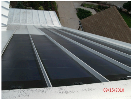
Figure 3: The steel is optimal for placing the PVLs in between its sections
