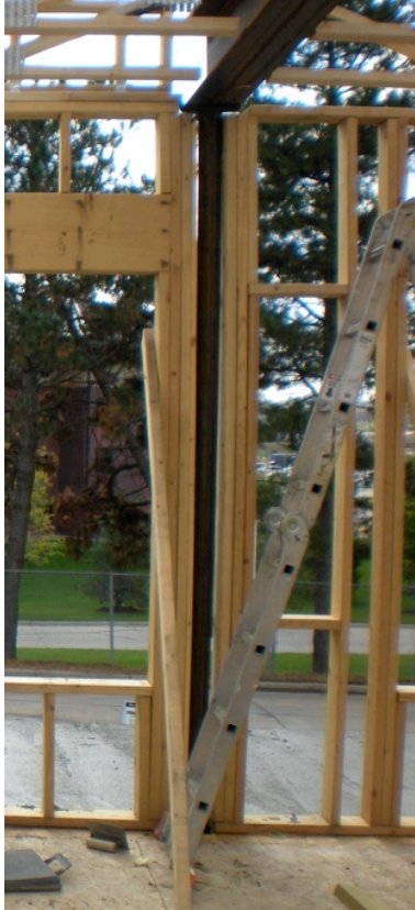
Figure 8: 24 inch spacing creates more room in wall cavities
