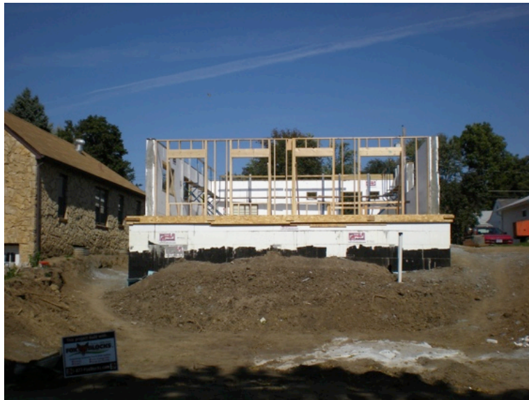
Figure 7: 2 x6 framed wall at 24 inch on center spacing
