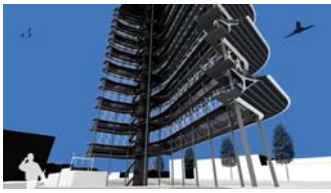
A central stair core connects the levels of the REI. Image courtesy of Chris Ford.
