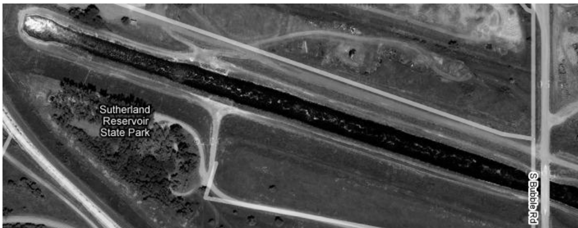
Figure 4.21 Aerial photograph of the outlet from Sutherland Reservoir. (Sutherland Reservoir outlet canal, maps.google.com, Aug, 2008)
