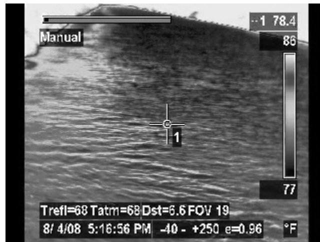
Figure 4.13 Upstream view of irrigation canal.
